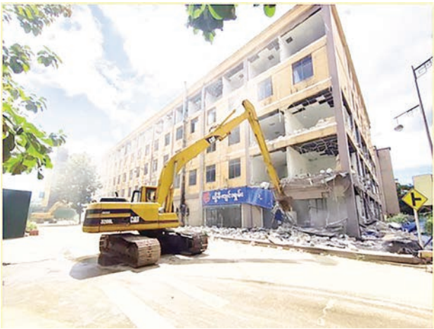
This image captures the demolition of scam-related structures in the Shwe Kokko area.
