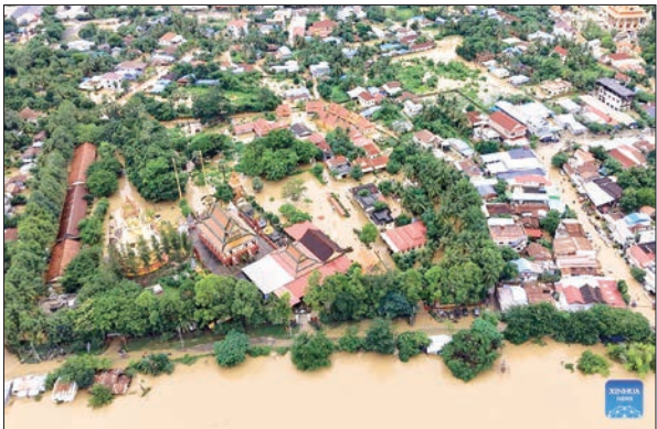
An aerial drone photo taken on 26 September 2026 shows a flooded area in Battambang City of Battambang Province, Cambodia. PHOTO: XINHUA
