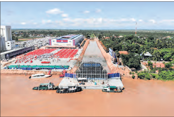
An aerial view shows the construction area after a groundbreaking ceremony of the Funan Techo Canal in Kandal province on 5 August 2024. PHOTO: AFP
