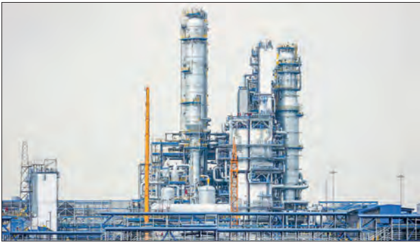
Gazprom’s Amur Gas Processing Plant, that extracts methane-associated gases from natural gas, as well as helium. PHOTO: SPUTNIK
