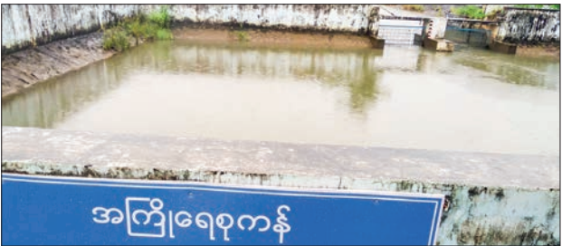
The Ngamoeyeik Water Treatment Plant (Nyaunghnapin).
