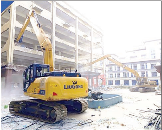
Systematic demolition of a scam-related five-storey building.
