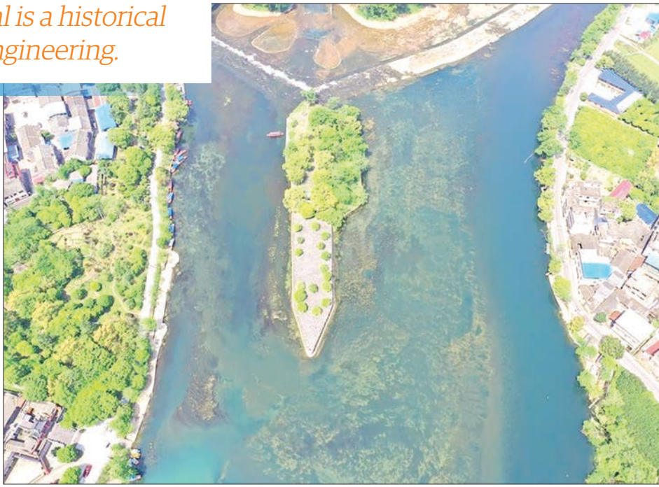
Aerial photo taken on 9 April 2022 shows Lingqu Canal in Xing'an County, south China's Guangxi Zhuang Autonomous Region. PHOTO: XINHUA
