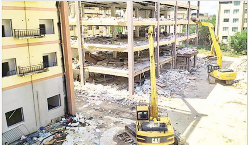
New image reveals the ongoing demolition of scam-related structures, buildings, and facilities in the Shwe Kokko area, Myawady, Kayin State.
