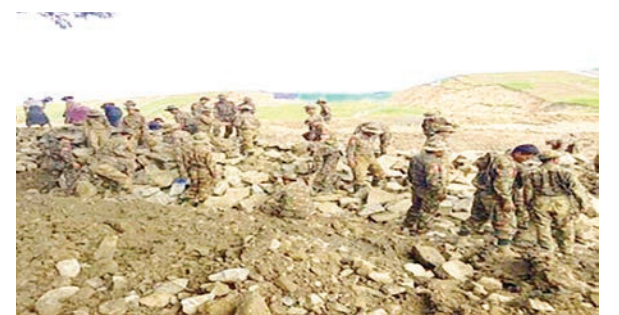
Tatmadaw members are seen at the work site of Ma Mya Dam in Myanaung, Ayeyawady Region.
