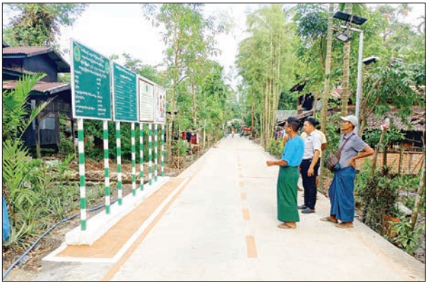
Officials inspect the completed concrete road in Myaungmya Township yesterday.
