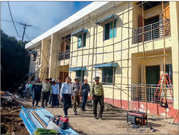
Officials inspect rehabilitation work in Falam Township.
