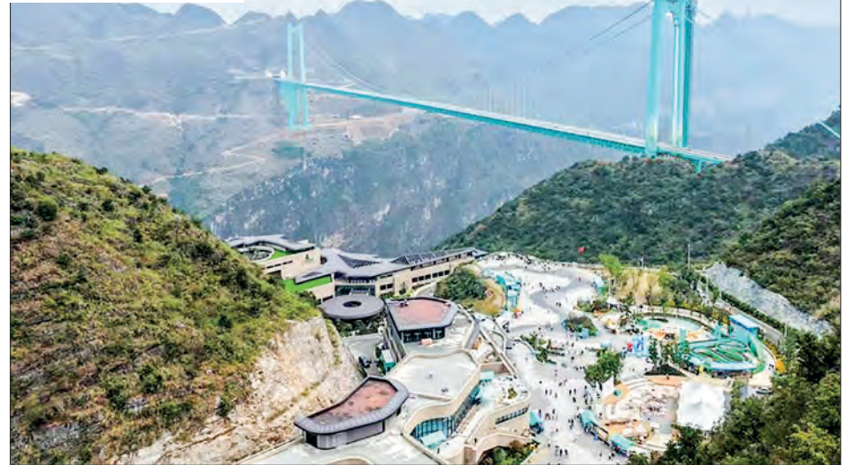
An aerial drone photo taken on 5 October 2026 shows the Huajiang Grand Canyon Bridge in southwest China’s Guizhou Province. PHOTO: XINHUA
