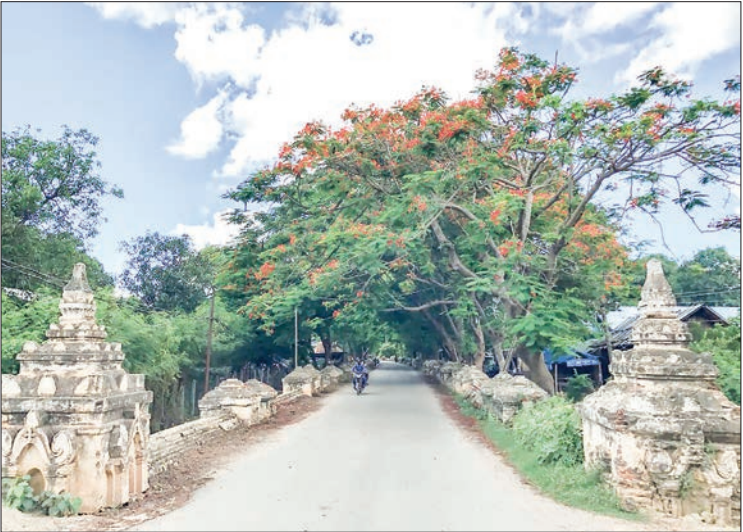
This photo features a section of the Maha Zeyapahta Bridge in Inwa.
