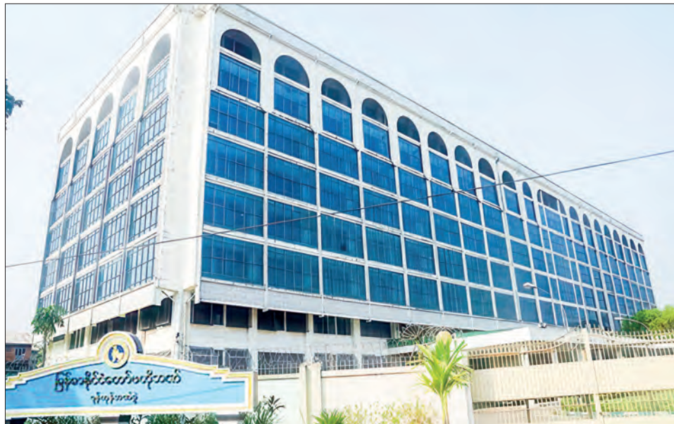
The front view of the Central Bank of Myanmar (CBM) in Yangon.
