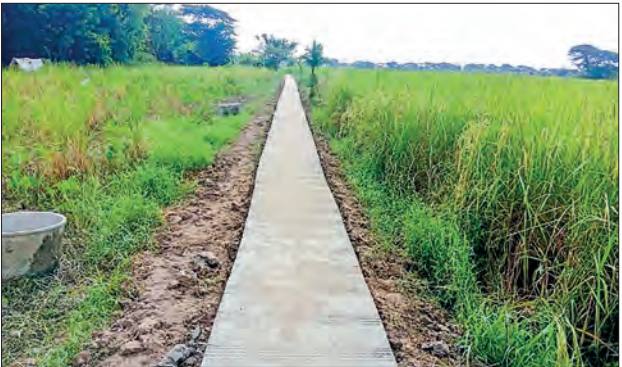
This image captures the concrete village road construction in Wakerma Township.
