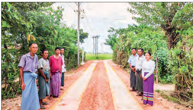
Officials are seen alongside the completed concrete wheel-track road in Gyobingauk Township.
