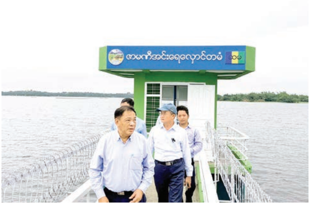
Officials inspect Zamani Inn Reservoir.
