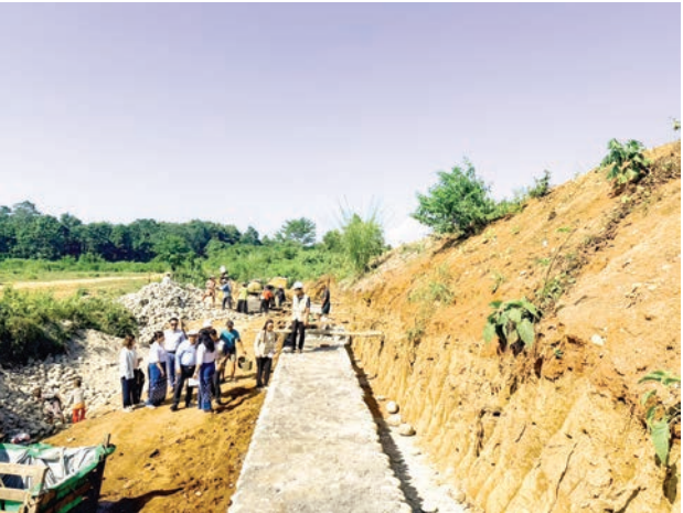
Officials oversee the construction of a retaining wall in Myitkyina Township.
