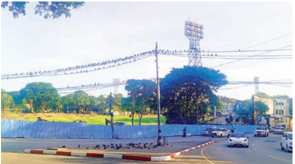
The image shows the progress of renovation works at the historic Aung San Stadium in downtown Yangon.
