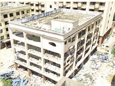
Systematic dismantling of a five-storey building in Shwe Kokko Phase II crackdown.
