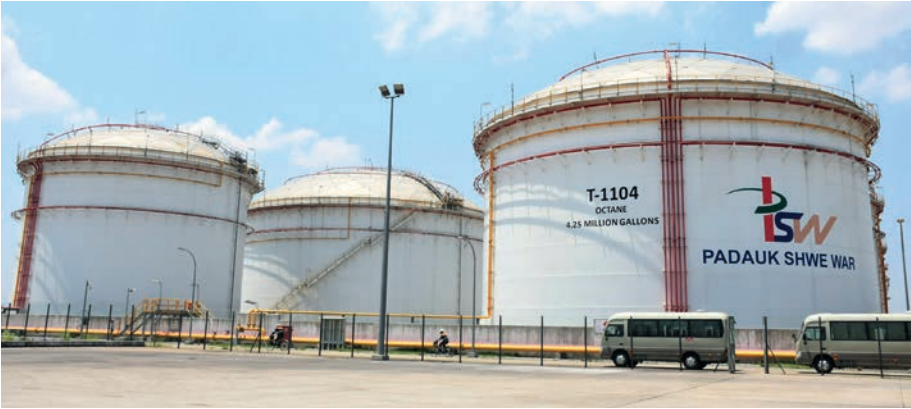
The image shows a row of Octane storage tanks.
