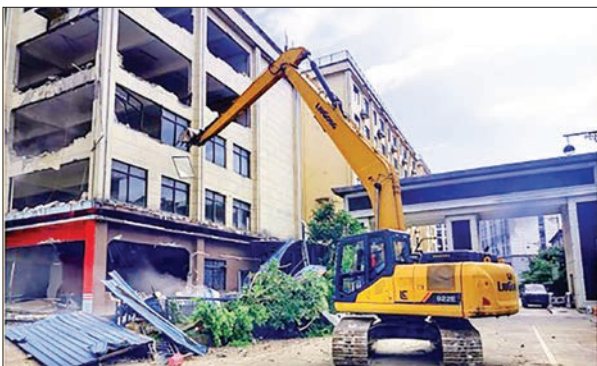
This image reveals part of the demolition in the Shwe Kokko area.
