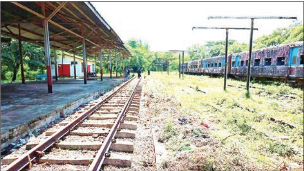
Officials are visiting Ye train station where renovations are underway.
