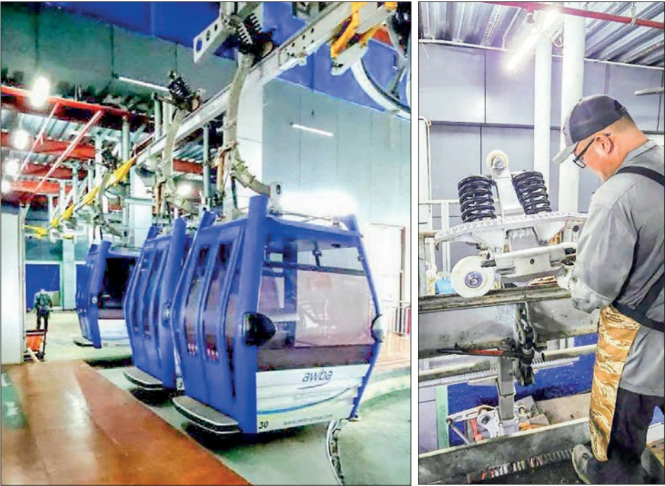
A technician repairs parts of cable cars to be ready for operations to transport pilgrims to Kyaiktiyo Pagoda.
