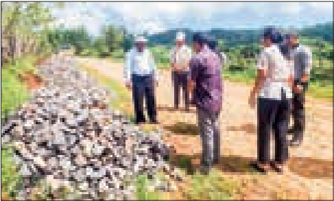
Officials inspect the progress of the paving the rural roads in Hopong and Hsihseng townships.
