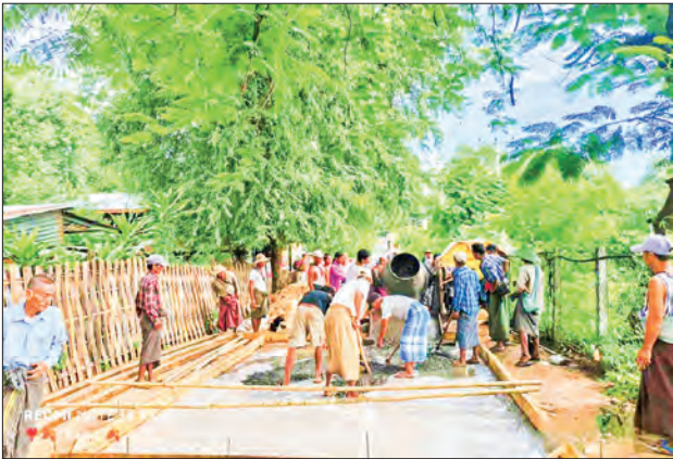
Officials oversee the village concrete road construction project in Kyaukpadaung Township.
