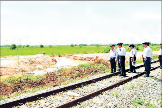
Officials inspect track-laying work on the new Toungoo bypass railway in Toungoo. the new railway connects line on the Mandalay side. — ASH/KZL
