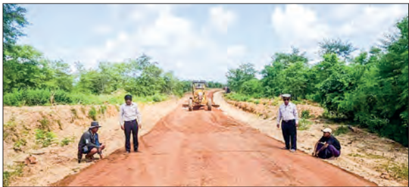
Officials oversee the road construction in Aunglan Township.
