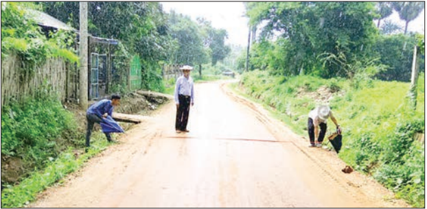
This image shows the completed road construction project in Yenangyoung Township.
