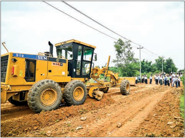
An operator uses a grader to widen the road around the Myitkyina Commodity Checkpoint.
