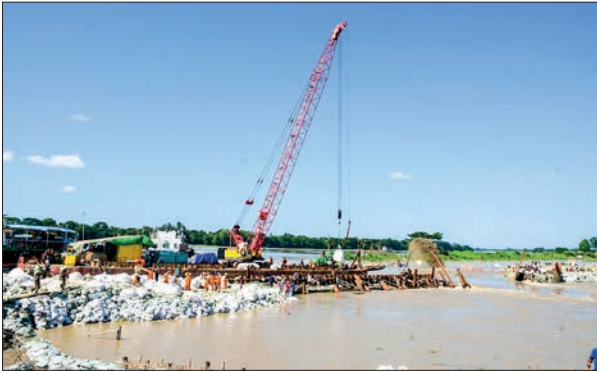
Flood recovery and repair works are underway with heavy machinery in Ayeyawady Region.
