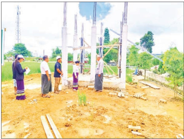
Officials inspect the ongoing water purification plant and water tank construction projects in Loikaw Township. THE Department of Rural Development, under the Ministry of Cooperatives and Rural Development, conducted a field inspection yesterday to review the progress of ongoing water purification plant and water tank construction projects in Pankan Village and Saikkwin 3 Village,
