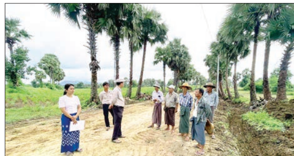
Officials inspect the ongoing road construction in Aunglan Township, Magway Region.
