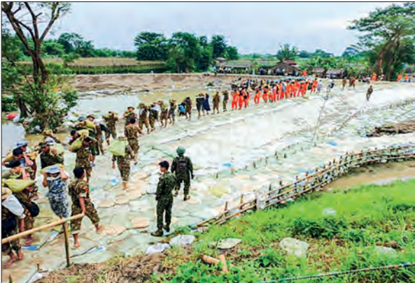
Collaborative efforts are underway to control embankment erosion in Nyaungdon Township.
