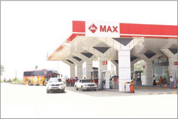
A fuel station selling oil by using Barcode, QR code scanning system.
