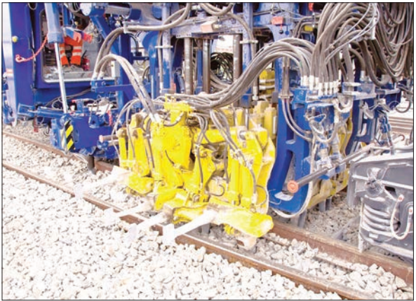
Lifting and packing railway track with the use of ALLTM machine.
