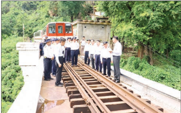
Union Minister U Mya Tun Oo inspects the repairs to the Nawngkhio-Gokteik railway. TRAIN services between PyinOoLwin and Gokteik will resume regularly from next Saturday after repairs to the Nawngkhio-Gokteik railway sec-
