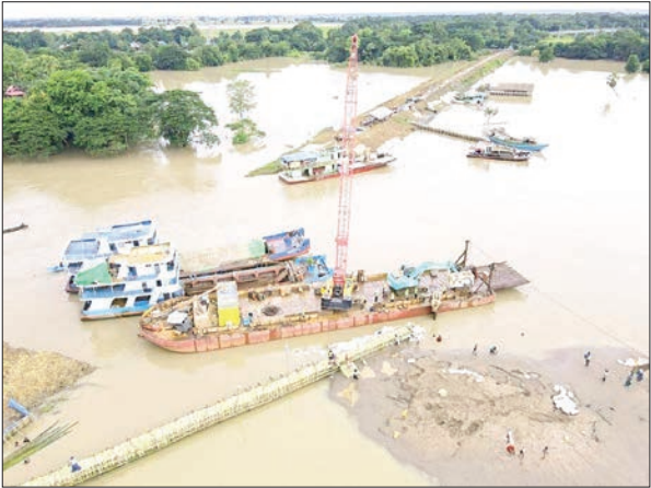
Accelerated repairs seal breach in Ngawun River embankment, Laymyethna Township, Ayeyawady Region.
