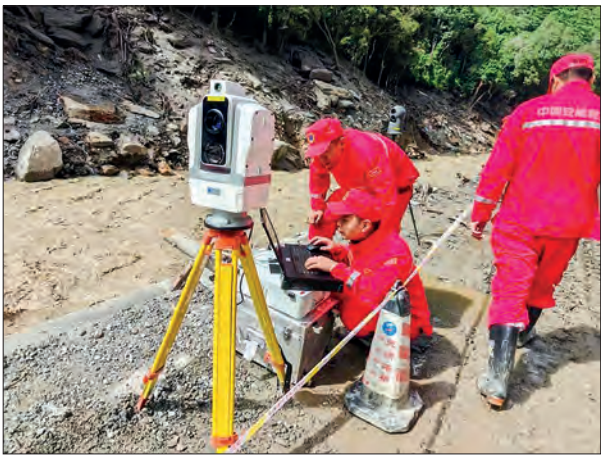
Rescuers use a laser-based AI monitoring device to dynamically monitor risks such as landslides and falling rocks at the mudslide-hit area in Gyirong County, southwest China’s Xizang Autonomous Region, 30 August 2026. PHOTO: XINHUA
