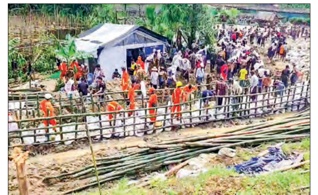
Tatmadaw and police personnel, social organizations and locals are carrying out to protect the damaged section to the Nyaungdonkyun embankment near Ganchaung Village, Nyaungdon Township.
