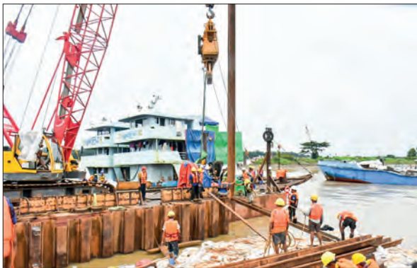
Officials and technicians use heavy machines to prevent erosion and block water inflows along the subsided section of the Ngawun embankment in Laymyethna Township.
