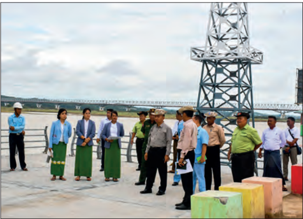
Officials inspect progress in building River View Point in Magway.
