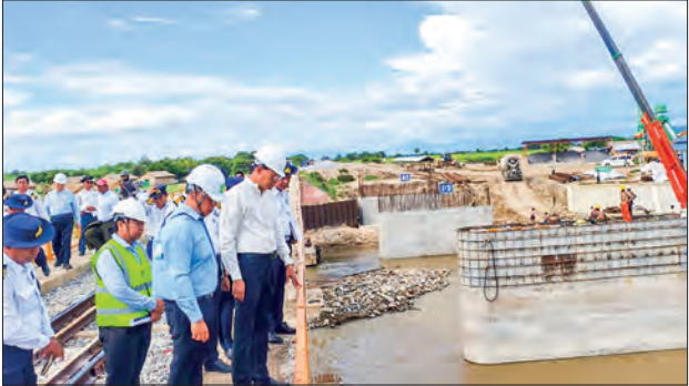
Union Minister U Mya Tun Oo oversees the construction site of the Samon Creek Bridge (Bridge No 691), on the Mandalay-Nay Pyi Taw railway line.
