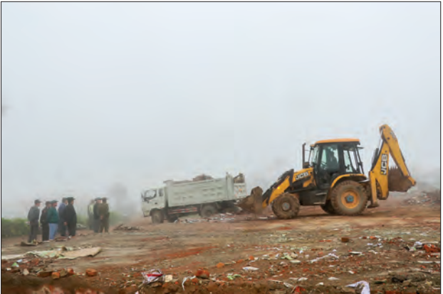
Residents with heavy machine are clearing debris at Falam People’s Hospital.
