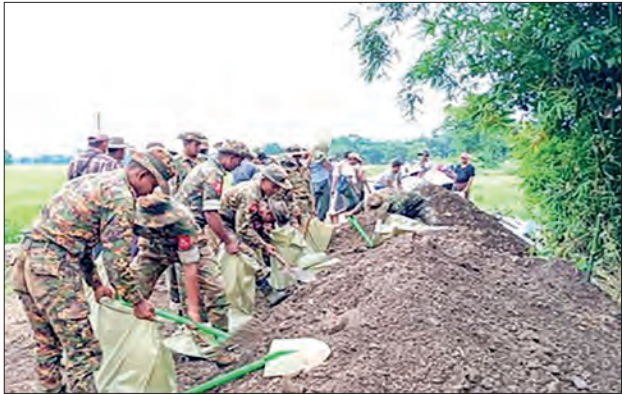
Flood recovery and repair works are underway in Ayeyawady Region.
