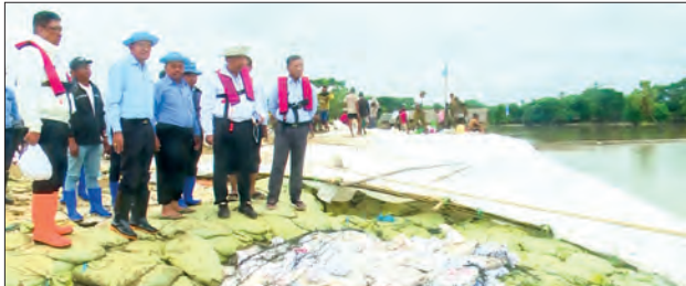
Deputy Minister U Bo Bo Kyaw and officials are pictured during their inspection tour in Laymyethna Township.
