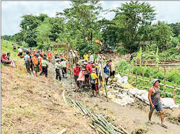
A collective effort is seen to protect the Nyaungdon embankment.
