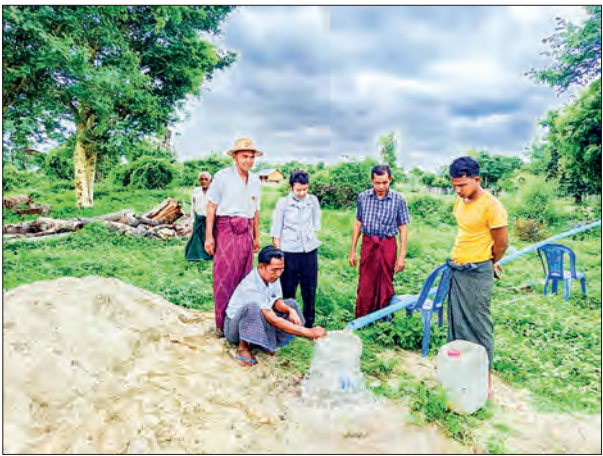
Officials oversee the water pump house construction project in Chauk Township in Magway Region.
