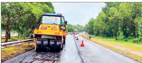
Construction of a tarred road is ongoing on the Yangon-Mandalay Expressway.
