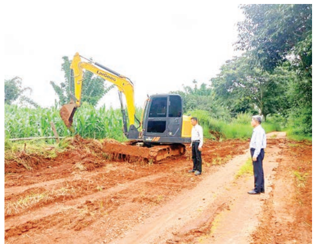
Officials inspect the construction site of a rural farm-to-market road project in Taunggyi Township.
