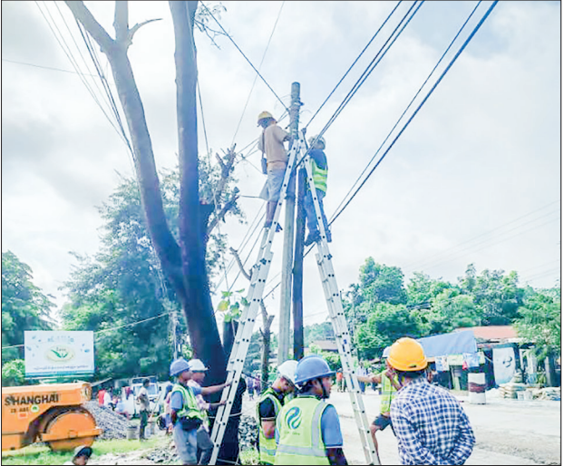
Technicians are installing cables of communications in Ayeyawady Region.
