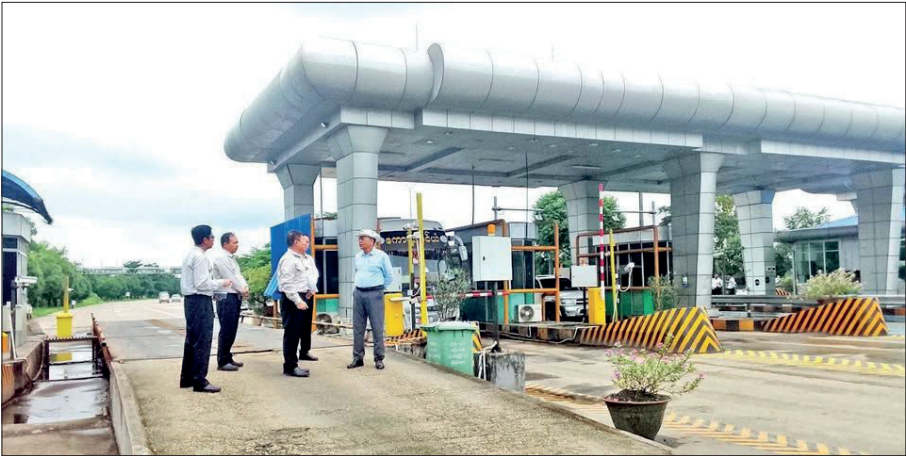
A checkpoint on the Yangon-Mandalay Expressway showcasing the trial of the Toll Pass RFID (Radio Frequency Identification Device) system.
