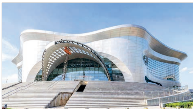
This photo taken on 22 July 2026 shows an exterior view of the joint customs and immigration inspection hall of the first cross-border ropeway linking China and Russia, in Heihe, northeast China’s Heilongjiang Province.
