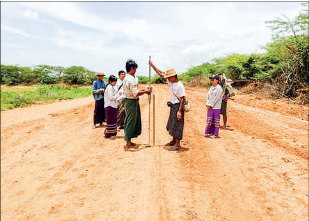
Officials and project committee members inspect progress of rural production road in Magway Township.
