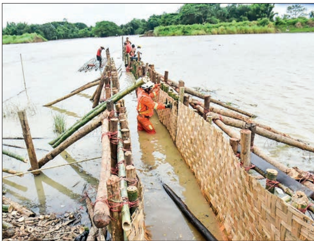
Volunteers are building barriers to prevent overflow of the Ngawun River in Laymyethna Township.
