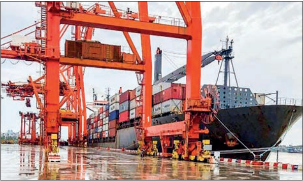
A merchant vessel is seen berthing alongside the Yangon Port.
