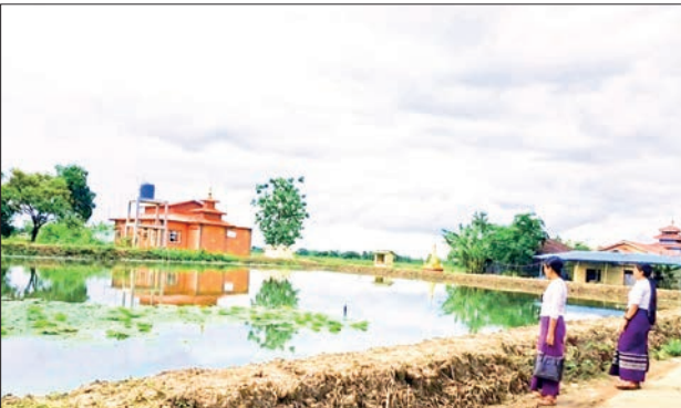
Officials oversee the completed water supply project in Dala Township, Yangon Region.
