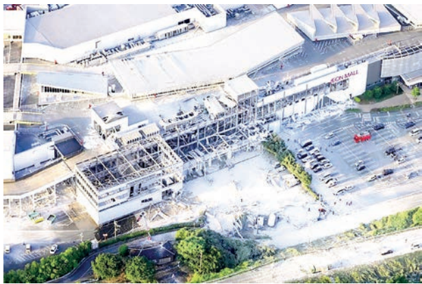
The Aeon Mall building in Kashima, Japan, after the earthquake Tuesday. PHOTO: KYODO
