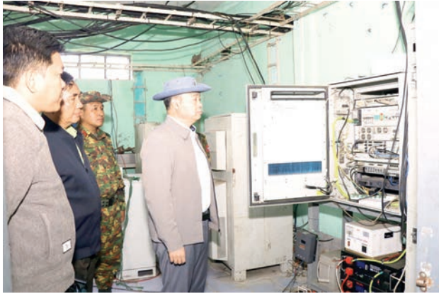
Deputy Minister Maj-Gen Kyaw Swa Oo inspects the installation of MEC TEL telephone lines at the Myanmar Posts and Telecommunications (MPT) at automatic exchange office in Falam, Chin State.
