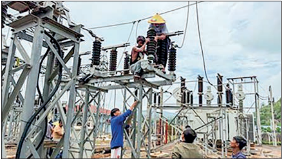
Employees from the Ministry of Electricity and Energy repair the electric power facilities at a power sub-station in Lashio.
