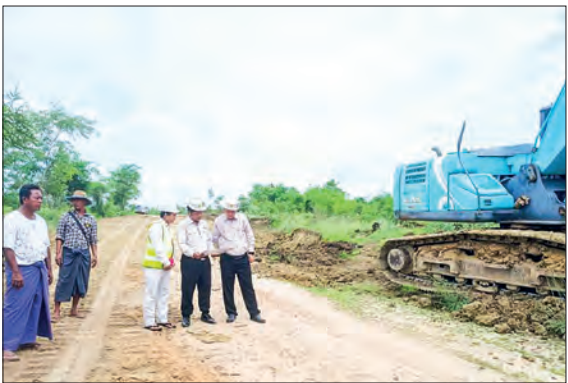
Officials inspect the village road construction project in Aunglan Township.
