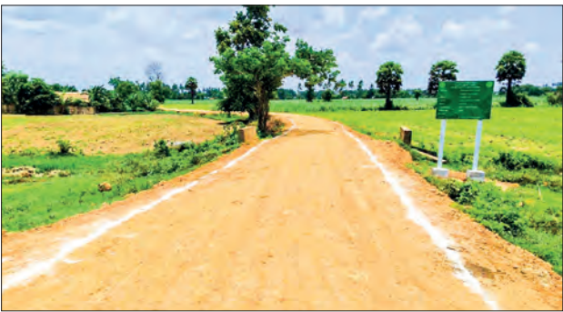
The completed road is seen in the picture.
