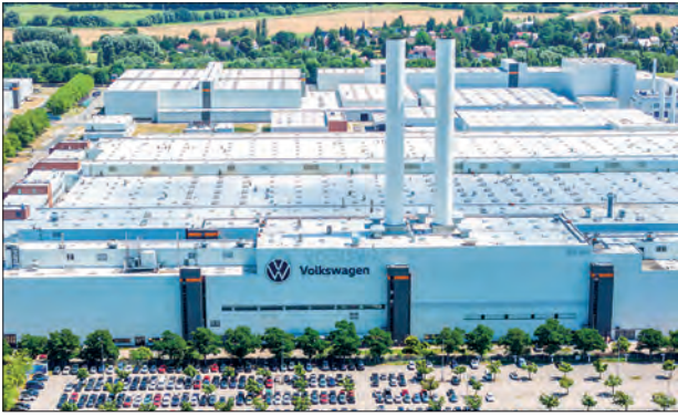
A general view at the Zwickau Volkswagen Plant on 9 July 2026 at the Zwickau, eastern Germany. PHOTO: AFP
