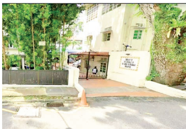
The facade of the Myanmar Embassy to Singapore.
