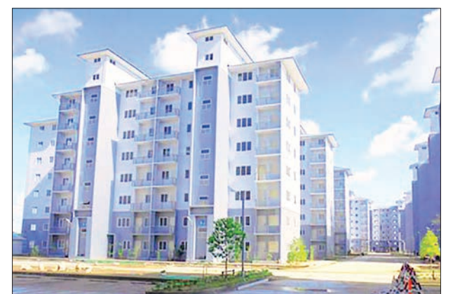
Allocated low-cost housing apartments in Shwepyitha.
