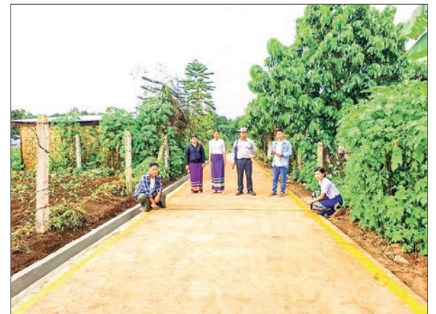
Officials inspect the completed village road concrete paving work in PyinOoLwin Township.
