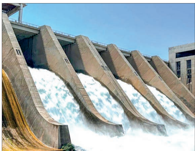
Water is discharged through a spillway gate at the Euphrates Dam in Raqqa province, Syria, 28 May 2026. PHOTO: XINHUA
