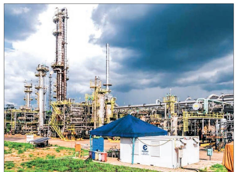
This photo taken on 16 October 2025 shows the production facilities of the Urucu Oil and Gas Production Field in the state of Amazonas, Brazil. PHOTO: XINHUA/FILE
