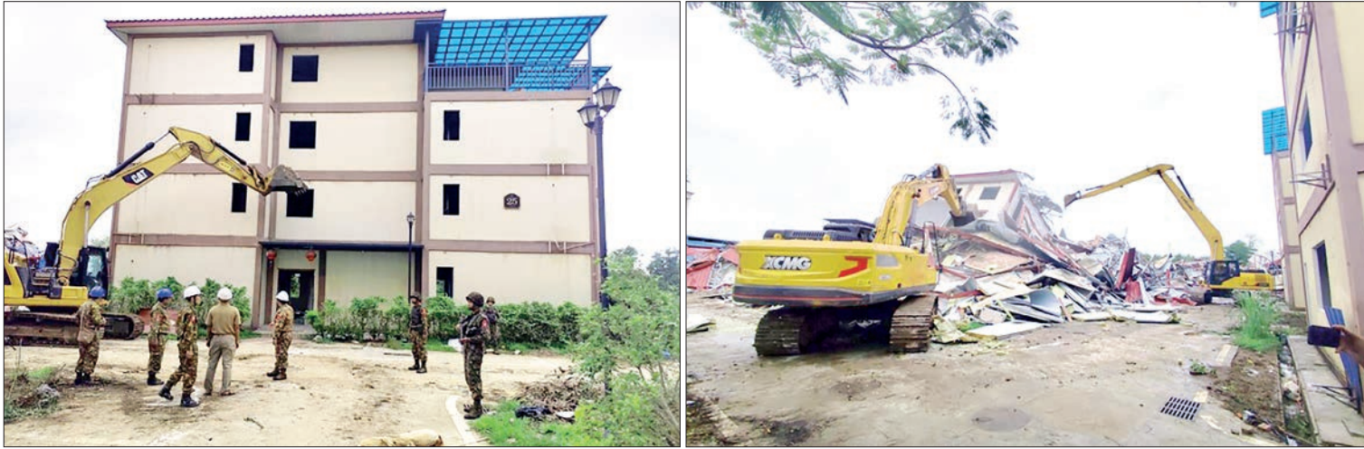
New images reveal the ongoing demolition of scam-related structures, buildings, and facilities in the Shwe Kokko area, Myawady, Kayin State.
