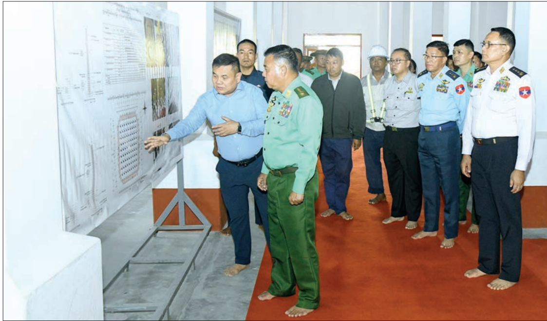
Defence Services Commander-in-Chief General Ye Win Oo is pictured inspecting repair work on religious edifices damaged by the Mandalay earthquake.
