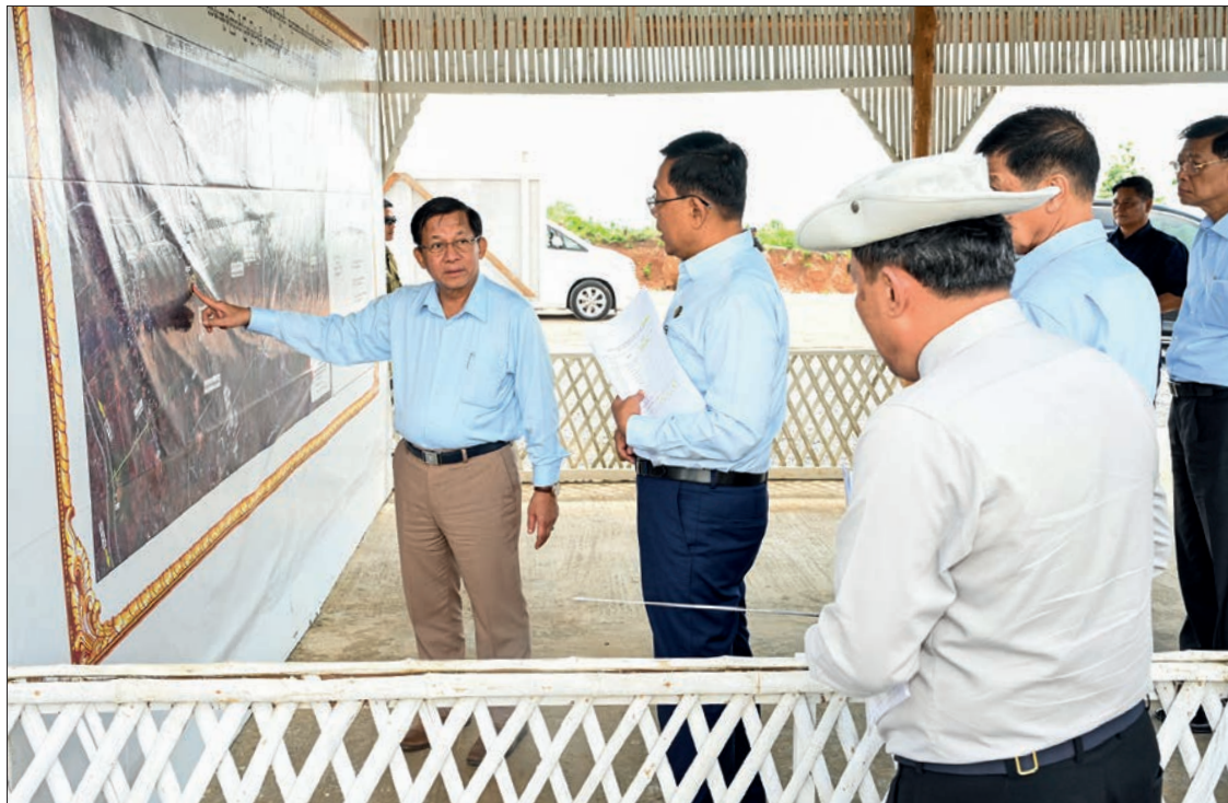
President U Min Aung Hlaing gives guidance over the construction of a new road leading to the Central Fire Services Training School from the Mandalay-Lashio Road.
