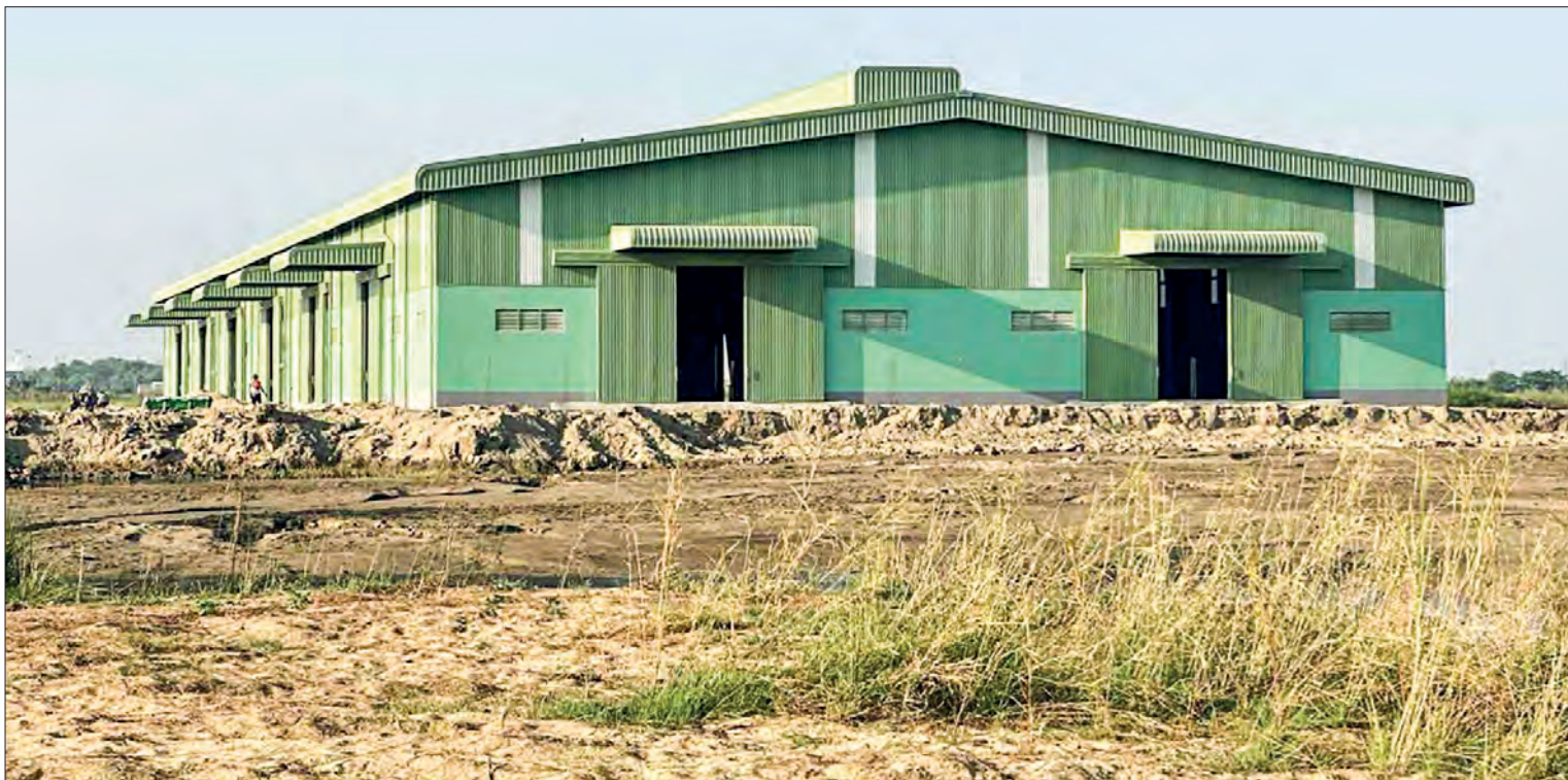
This photo captures a warehouse under construction.
