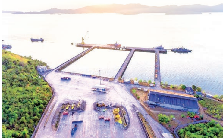
The image shows an aerial view of Ranong Port in Thailand. PHOTO: PIX FOR VISUAL PURPOSE/ LOGISTICS MANAGER
