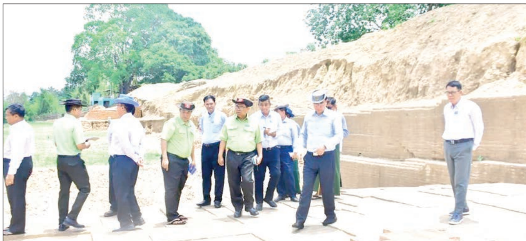
This photo shows officials inspecting construction work.
