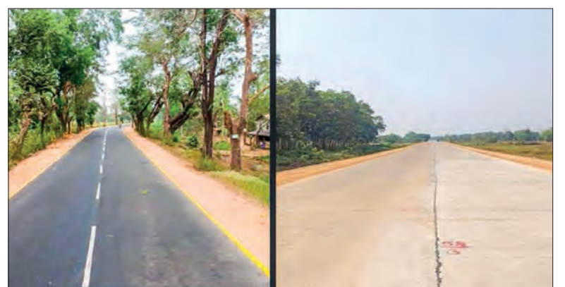
Images show the Yangon-Pathein road sections after asphalt overlay and concrete paving work.
