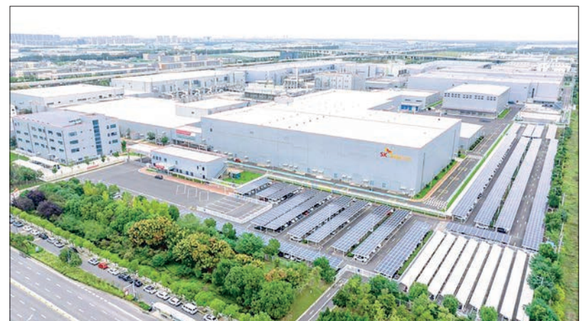
This aerial drone photo shows a view of a new energy battery production base of South Korean EV battery maker SK On Jiangsu Co Ltd in Yancheng, east China's Jiangsu Province, 16 October 2025. PHOTO: XINHUA
