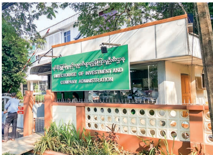
The facade view of the DICA office in Yangon.
